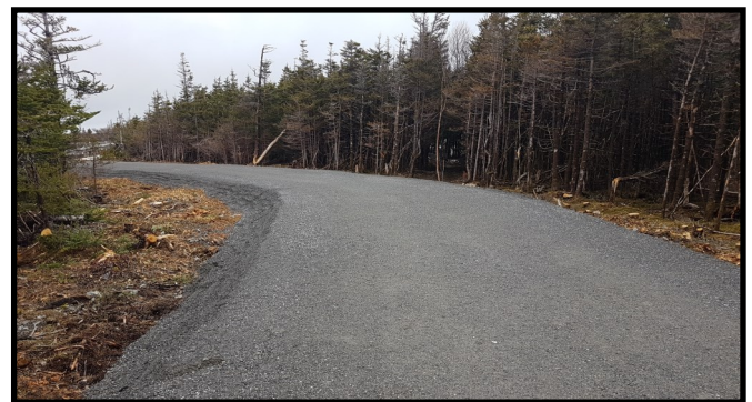
Below: A wider trail allows for multi-use activities such as bicycling. It also allows for a better emergency medical response.
